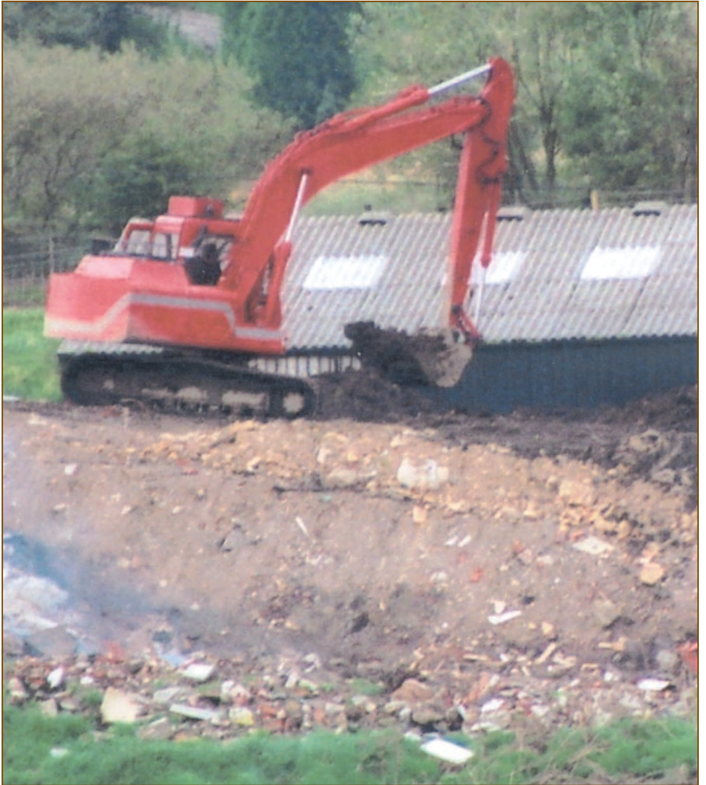
Photograph of excavation on neighbouring land (paragraph 51).
